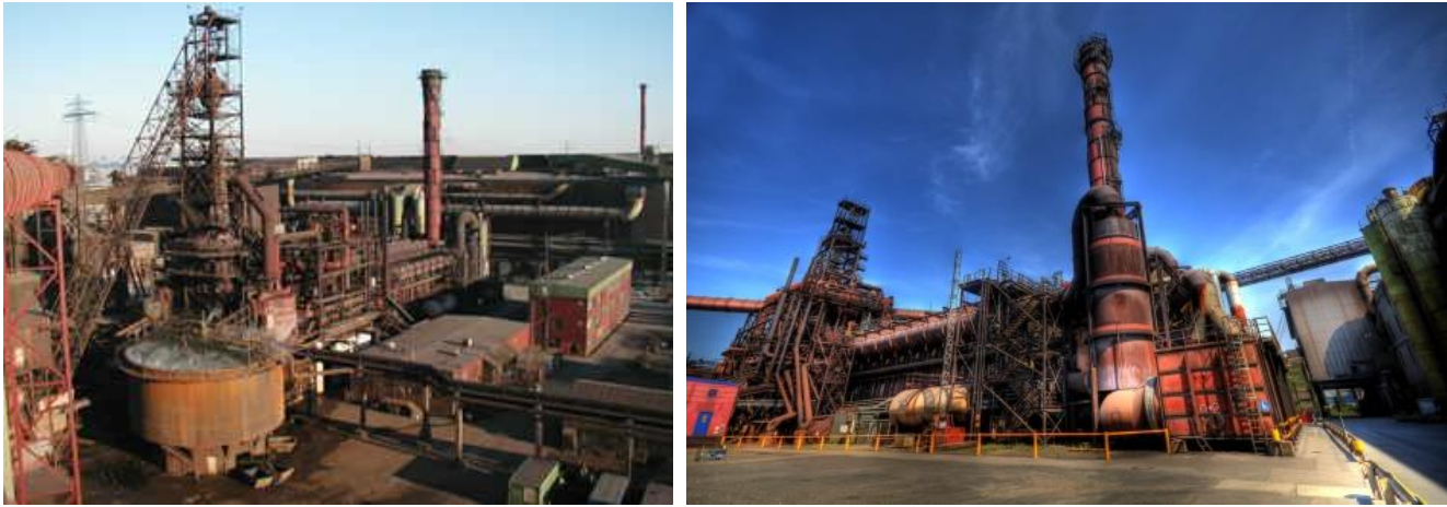
Figure 10: Midrex® DR plant at ArcelorMittal Hamburg AG
