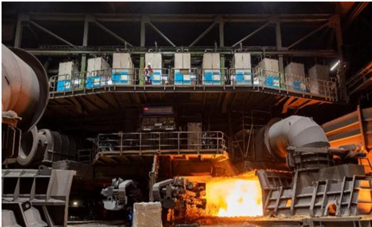
Figure 3: Image of Schwelgern BF1 SIP boxes, located on a platform above the tuyere level
