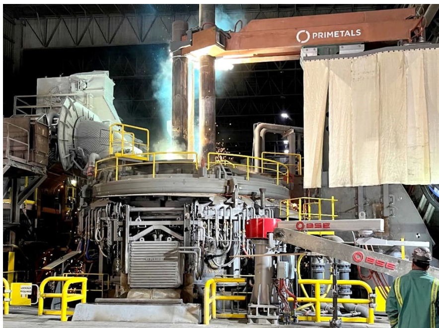
The 118-ton EAF, revamped by Primetals Technologies, at the first heat.
